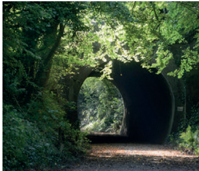
West Dean Tunnel, Centurion Way © SDNPA
